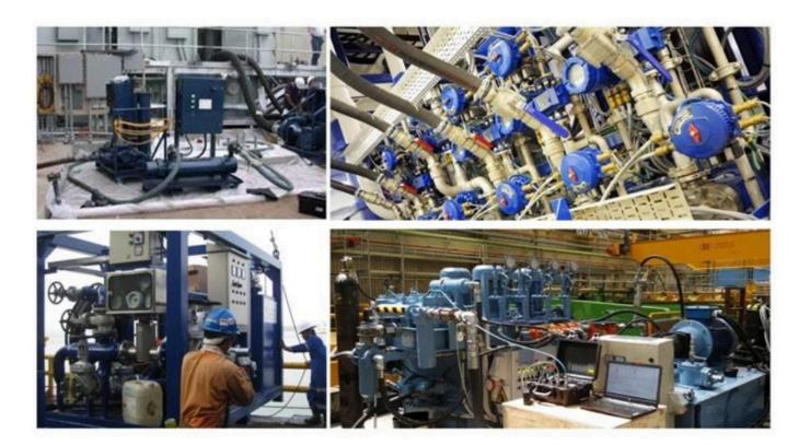
Flushing is a process which is done to clear any contaminants present in the pipe and oil after installation. The sole purpose of this process is to avoid damage caused by contaminants/dirt's to the end using equipment. The pipes are cleaned by creating a turbulent flow in the system and passing them through filters until the desired cleanliness value is obtained.
