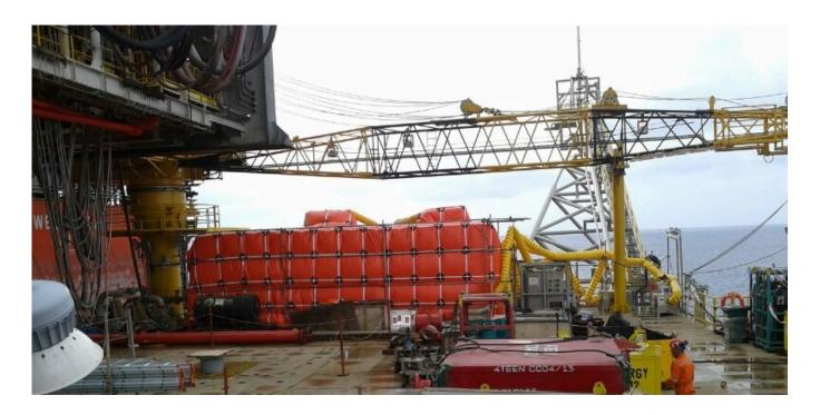
The WICH System is designed based on flexibility in mind, which helps facilitate hot work better. It comes in versatile designs, various sizes, is able to fit in any space and each part is easily transported. The use of scaffolding and pliable covering alsoallow the system to be builtaroundpillars other obstacles
