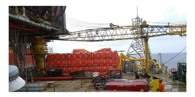
The WICH System is designed based on flexibility in mind, which helps facilitate hot work better. It comes in versatile designs, various sizes, is able to fit in any space and each part is easily transported. The use of scaffolding and pliable covering also allow the system to be builtaround pillars and other obstacles
