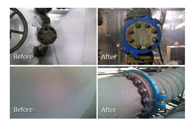
PT Pradita Puncak Sarana provides non-destructive, online, stream leak repair services for process, team, water, and air leaks. These repair services are made at temperatures ranging from cryogenic to 700 deg C, and pressures from vacuum to 200 bars. From low-cost banding or open wire from marrow gap flanges and bonnets to solutions based on ring clamps or box enclosures, we provide alternatives.
